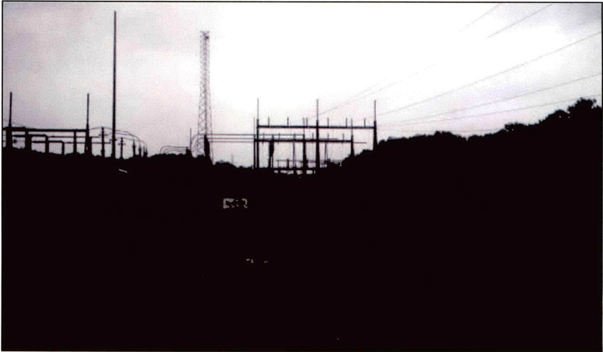
Figure 3-p. Location #15—Big Rivers Coleman Extra High Voltage (EHV) Substation.
