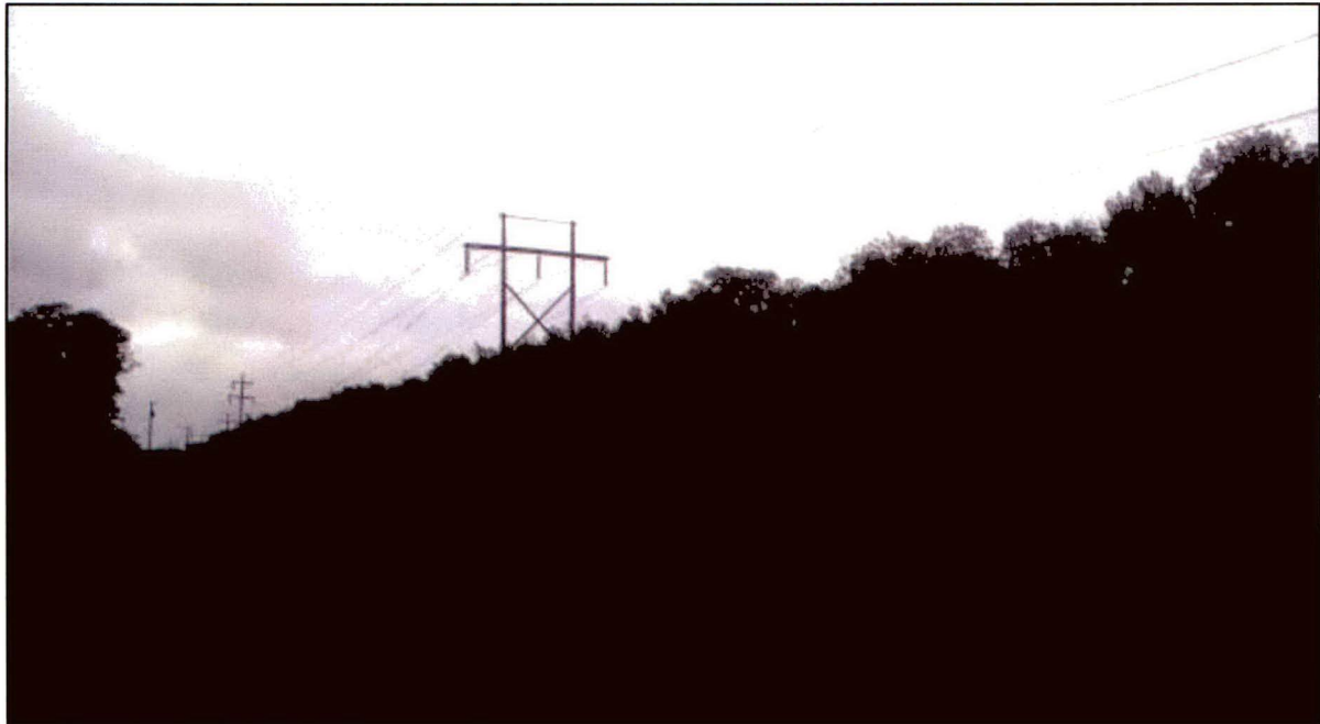
Figure 3-k. Location #10—View of Big Rivers' transmission lines south of the Seaboard Railroad track. Looking east along the utility right-of-way, the tree line (to the right) is the northern edge of a large, contiguous forest block that extends eastward toward Adair Road.
